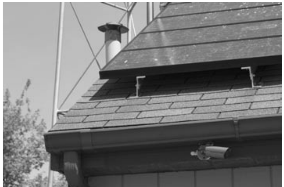
Solar panels on the roof of the building that houses Stelle’s solar-powered telephone company are raised about six inches to allow air to circulate under the panels.
