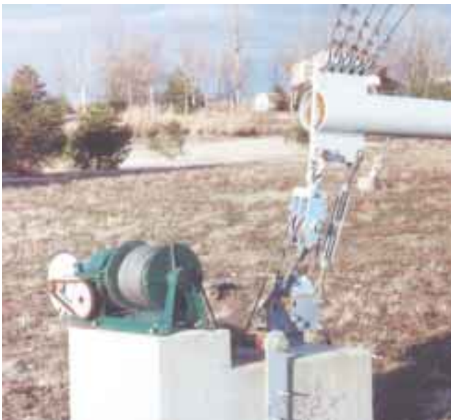
The winch, with block and tackle, at the gin pole.
